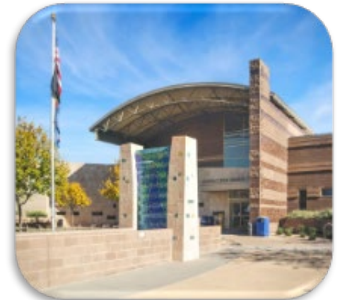
Solar at Existing Town Facilities
