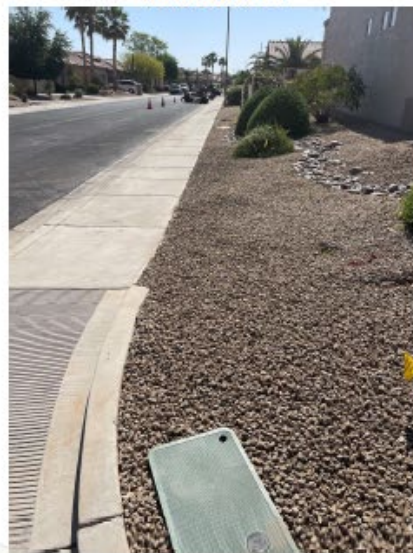
Completed HH At the edge Marks cleaned
