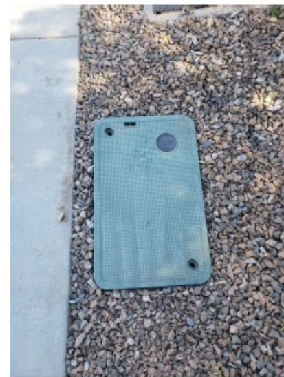
Completed HH Along ROW
