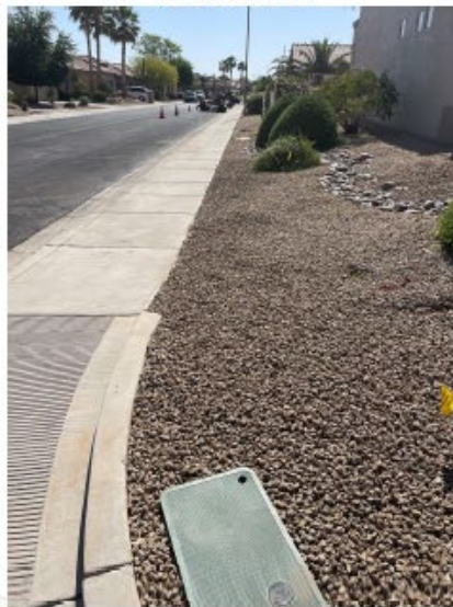
Completed HH At the edge Marks cleaned
