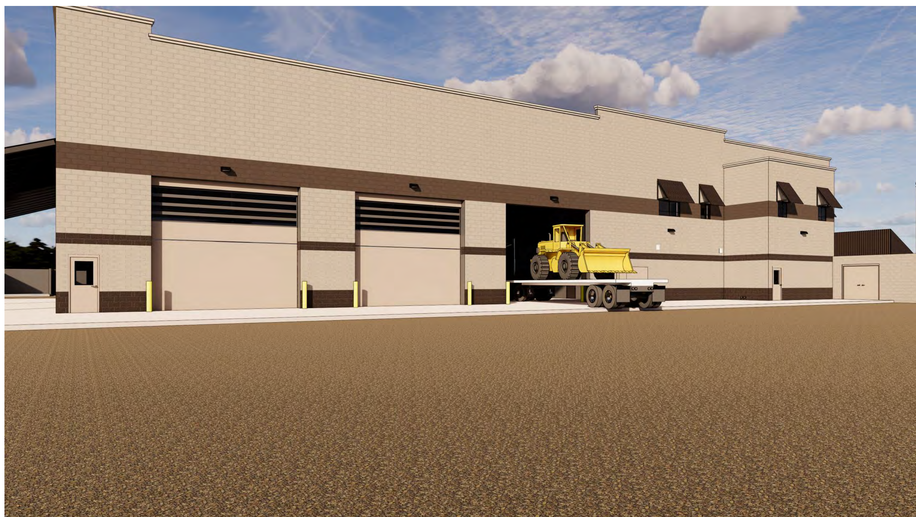
South Face of the Shop
