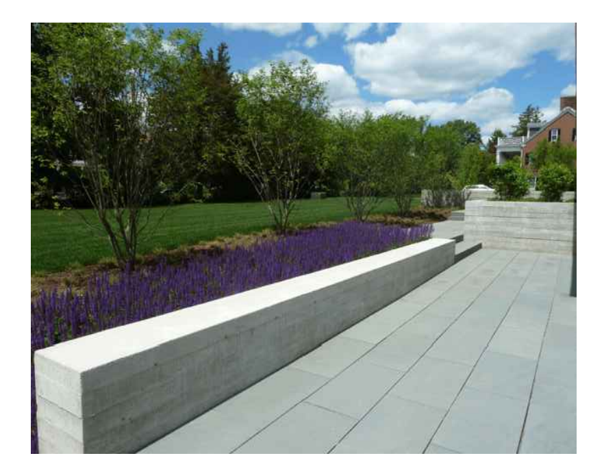
Seatwall Cast In Place Concrete
