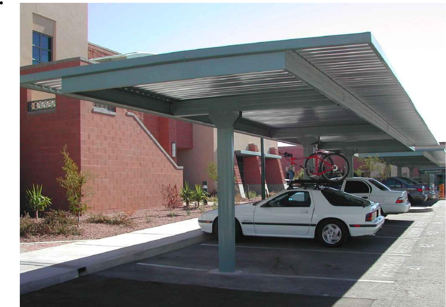
SEMI-CANTILEVERED CARPORT NOTE: IMAGE FOR REFERENCE ONLY
