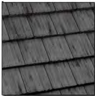
Roof Mfg: Eagle Roofing Ponderosa 5503 Sierra Madre
