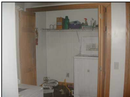
FIGURE 3-25: Laundry Room Fire Extinguished by One Sprinkler
