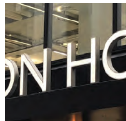
Channel Letter Mounted on Canopy Face OR Halo Illuminated with Hidden Raceway
