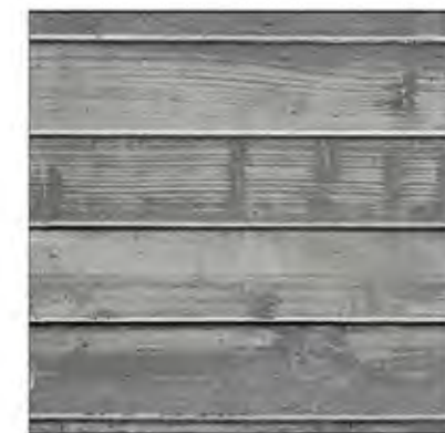
PC: Precast Concrete "Natural" CC: Board Formed Concrete "Natural"
