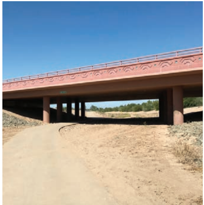
Sonoqui Wash Trail Underpass at Chandler Heights Road
