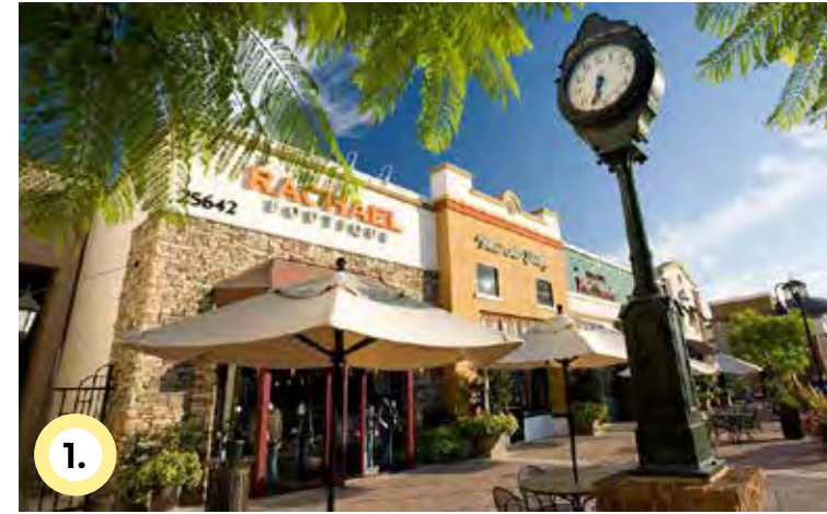
1. Doors should be easily readable and recognizable, but not overly large. Use vertically oriented doors and architectural elements to enhance the entry and provide consistent horizontal spacing between windows.
