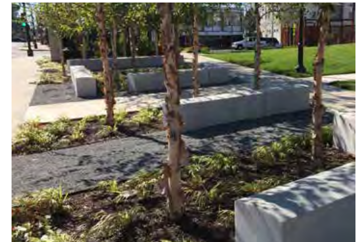
Retention walls can be designed as seating areas in the public realm.
