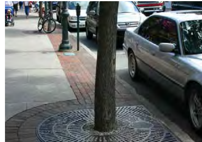
NOT THIS Tree grates with not sufficient space for growing trees, can become problem overtime.
