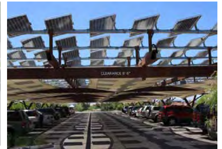
Provide solar panels over parking stalls when possible to create shade and sustainable surface.
