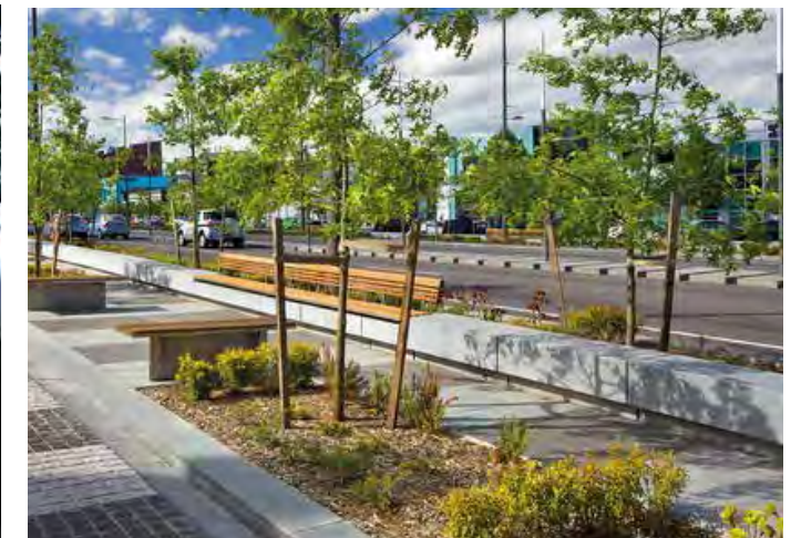
THIS Bio retentions are shallow depressions used in urban conditions where subsoils are porous and allow infiltration into the subgrade.
