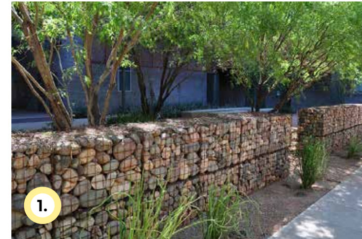
Low walls help define landscape areas, spatial transitions, drainage, and integration of different uses.
