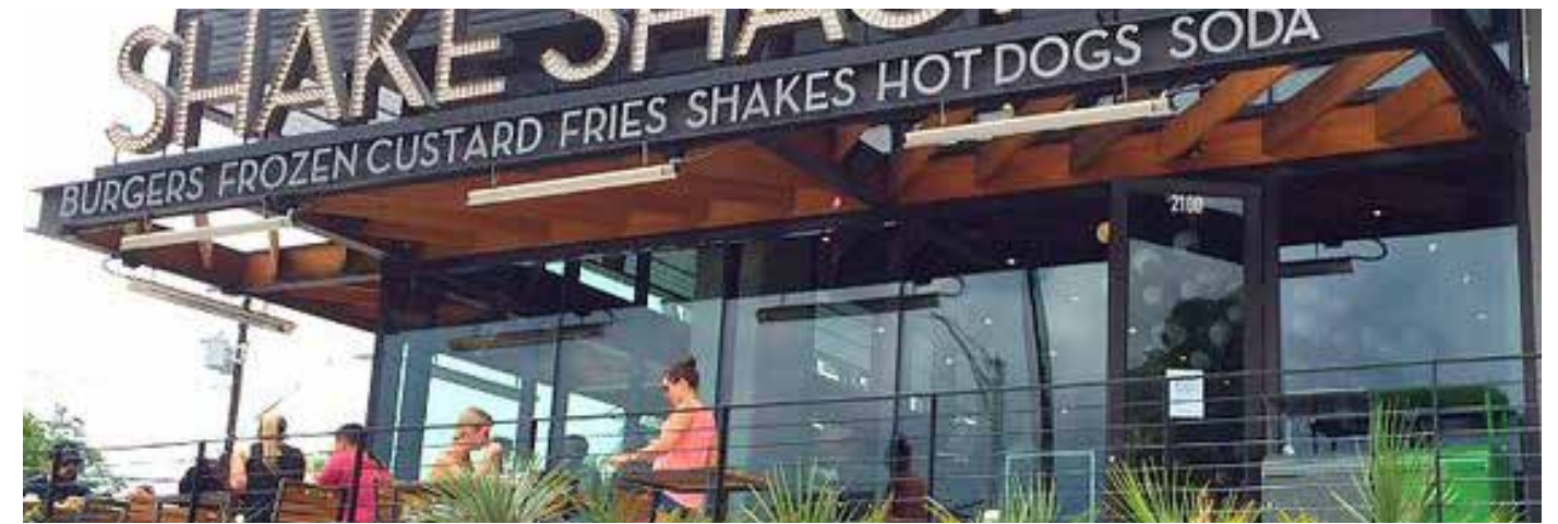
The awning sign is a horizontal, projecting object. This category includes traditional awning forms as well as contemporary, flat projections.
