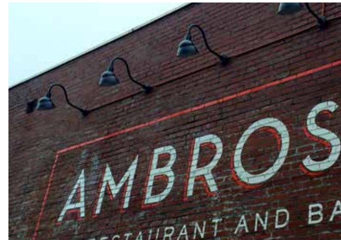
Select light fixtures that are similar in style to buildings along and direct light down towards building face.
