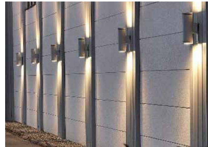
Light fixtures can be architecturally placed to enhance special building shapes.
