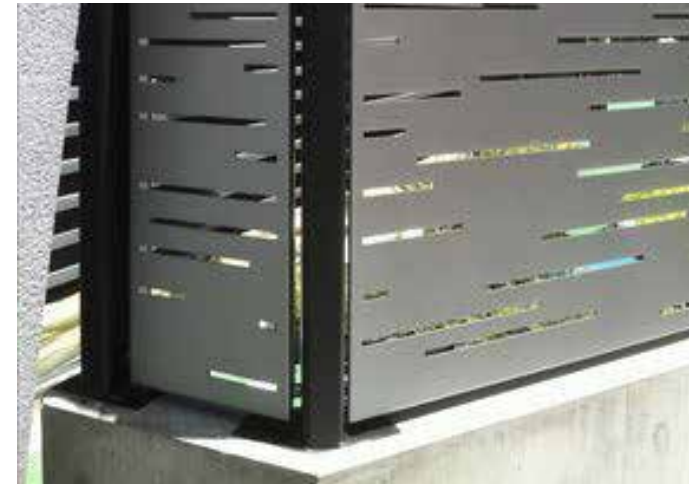
Utilities screens are effective making large boxes or transformers almost invisible.
