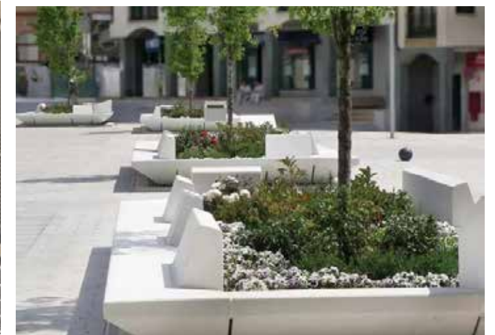
THIS Above ground rainwater harvesting systems capture stormwater runoff, and stores the water for later use.
