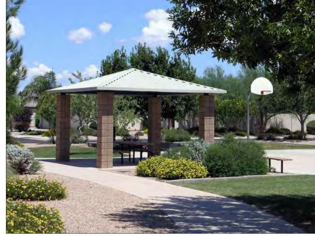
LARGE RAMADA (2 LOCATIONS) MANUFACTURER: CLASSIC RECREATION SYSTEM, INC. MODEL #: 24' X 24' DENVER WITH STANDING SEAM ROOF ROOF COLOR: "WEATHERED COPPER"
