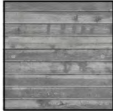
BOARD FORMED CONCRETE GRAY CONCRETE WITH 2x6 ROUGH SAWN WOOD FRAME TO ACHIEVE LOOK
