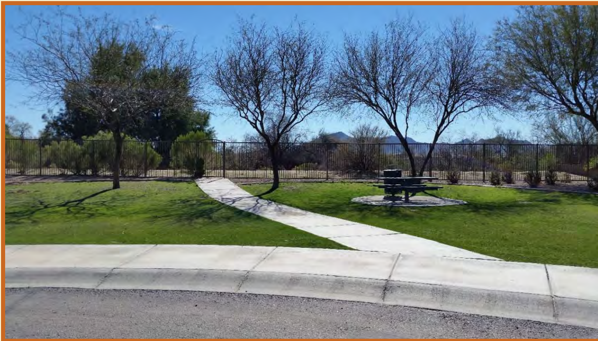
Partially completed connection to the future Queen Creek Trail at the end of East Pecan Drive
