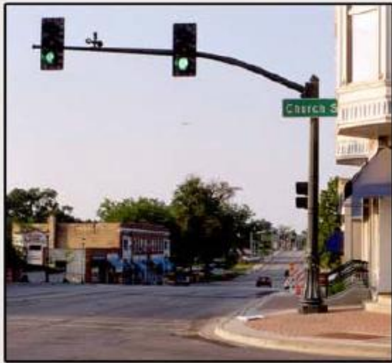
Traffic Signal Lighting
