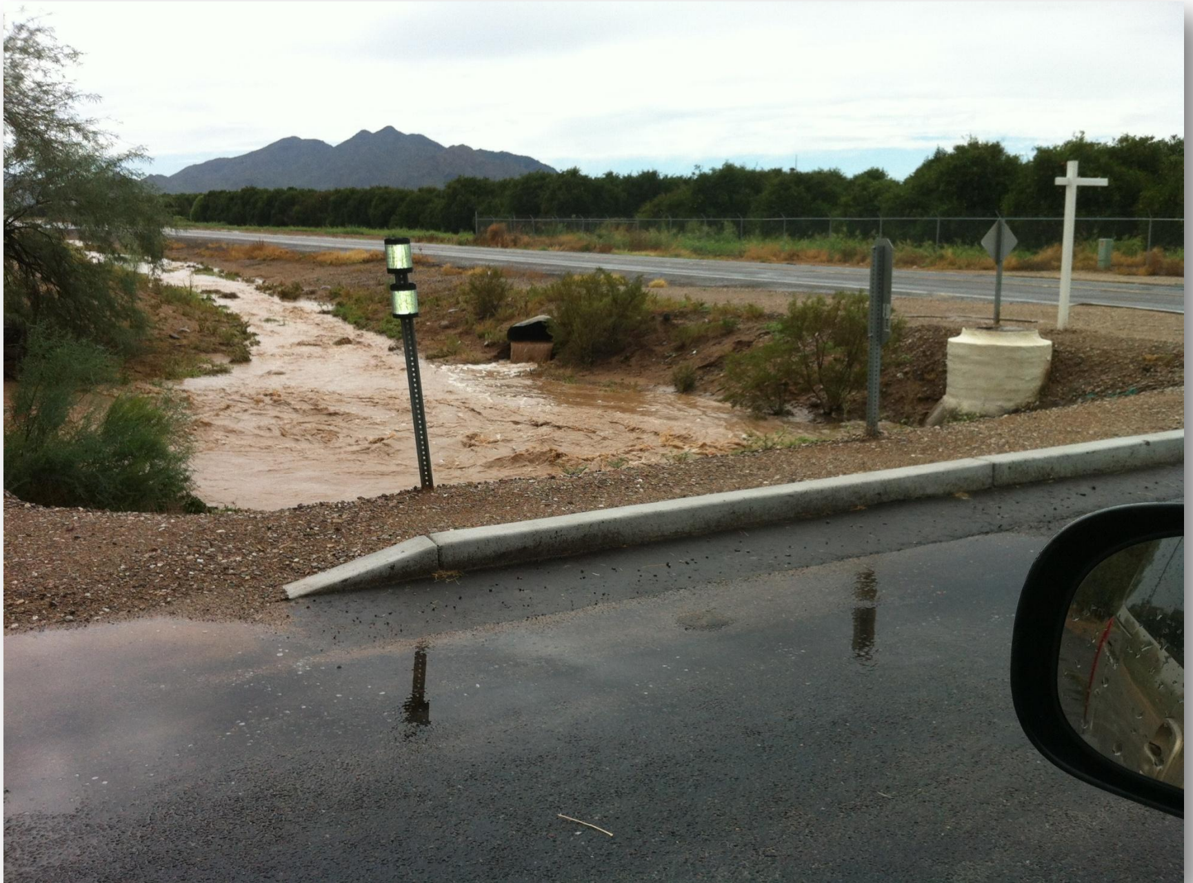
Power Road Channel at Cloud Road
