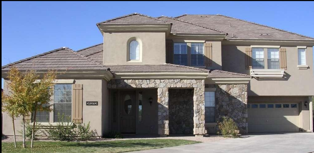
Not This: Too many different proportions are used on this façade.
