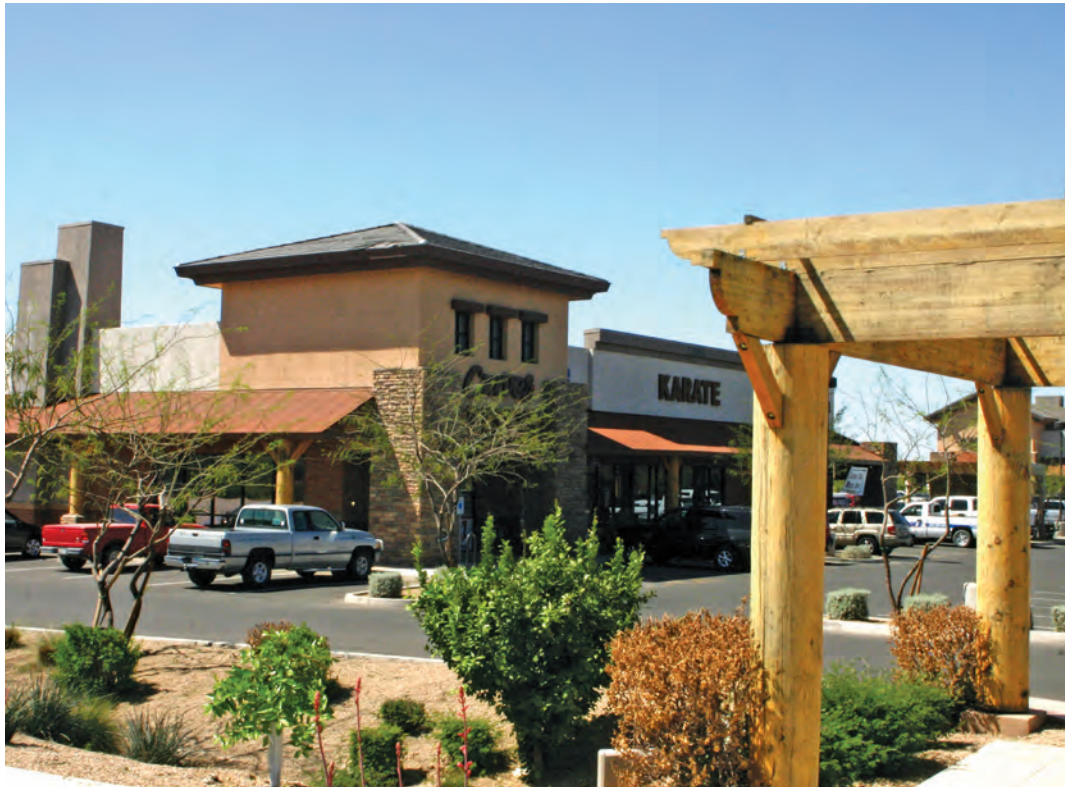
The town is composed of a variety of agricultural, residential, and commercial land uses. Recent retail uses have employed high-quality architectural features that embody the historic feel of the Southwest.
